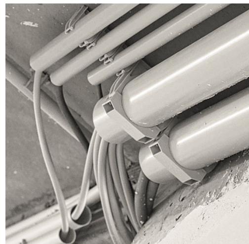
With the UVB, even tubes with heavy cable bundles are held securely in the EC.
