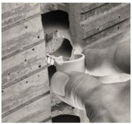
Simply brilliant: the integrated nib on the interior side of the clip enables the pipe to tense between the two clips for easier cable insertion.
