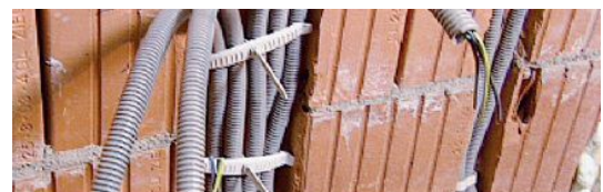
With the TB in two sizes, Schnabl has in combination with the TA a system for all requirements - on or under plasterboard
