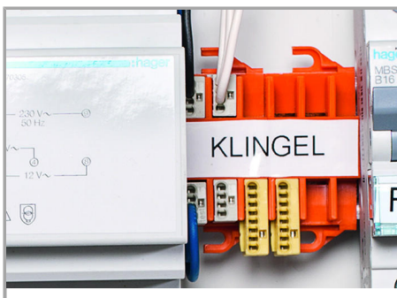
Example of a residential door bell application
