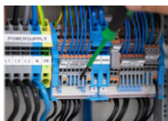
Tool-operated N-disconnect slide link
