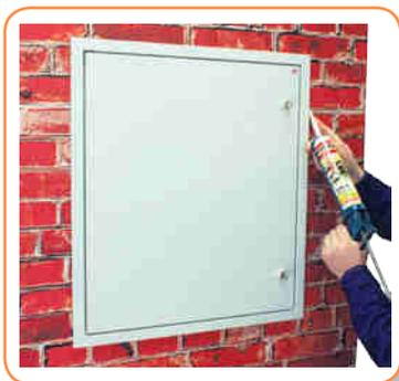
For achieve proper degree of protection, space between door frame and the wall should be sealed by silicone sealant.
