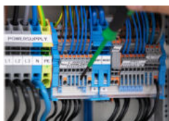
Tool-operated N-disconnect slide link
