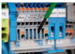
Tool-operated N-disconnect slide link
