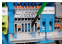
Tool-operated N-disconnect slide link
