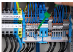
Tool-operated N-disconnect slide link
