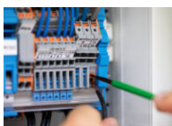
Conductor termination
